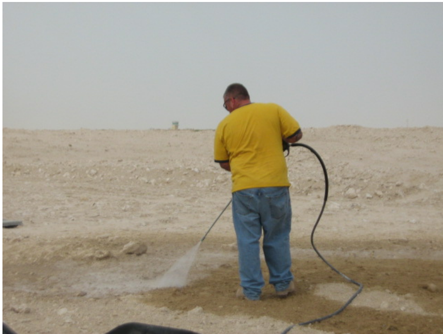
Figure 3 Spraying water on the Micro-Blaze ® -treated soil contamination
