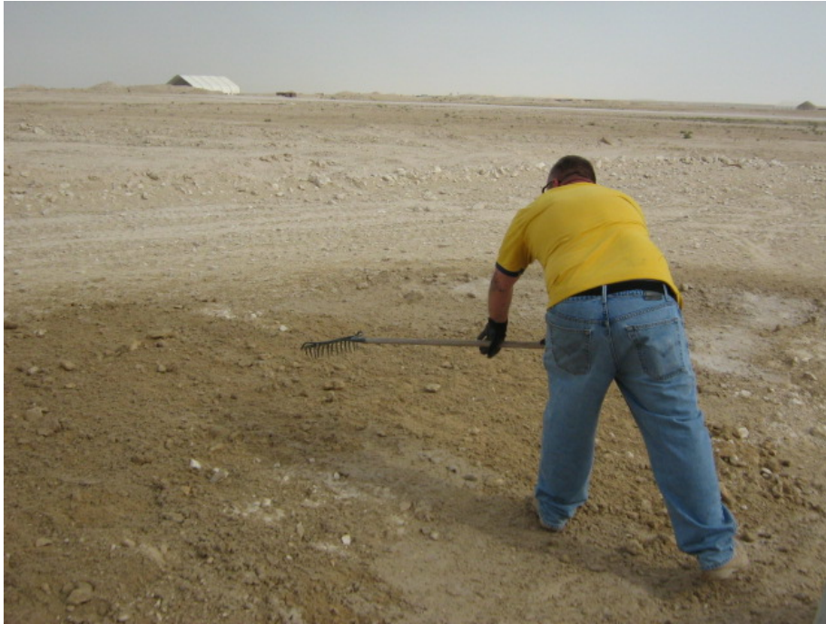
Figure 2 Tilling the soil to expose deeper fuel contaminated soil to Micro-Blaze ®
